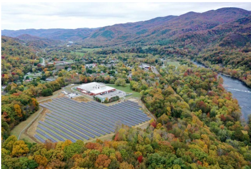
Hot Springs Microgrid - Duke Energy
