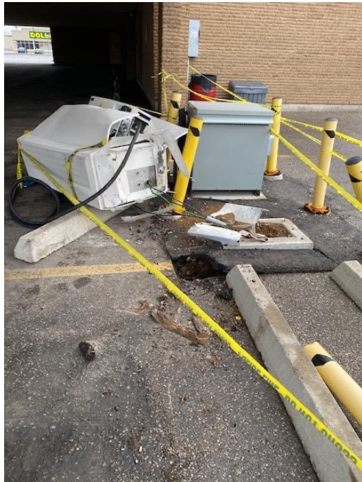
Charger without bollards vulnerable to being struck by a vehicle
