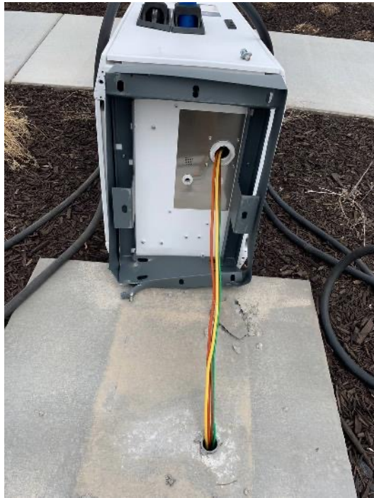
Charger without bollards vulnerable to being struck by a vehicle
